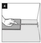
At the end of the first row, leave an expan sion gap of % to the wall an length of the last plank to fit.
